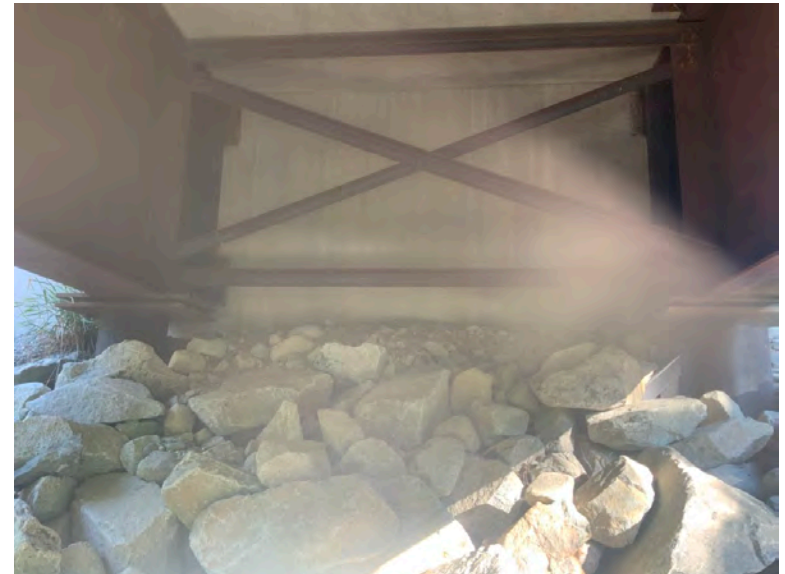
Left Bank Abutment when facing downstream
