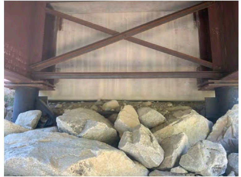
Right Bank Abutment when facing downstream
