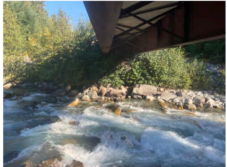
Left Bank Abutment when facing downstream
