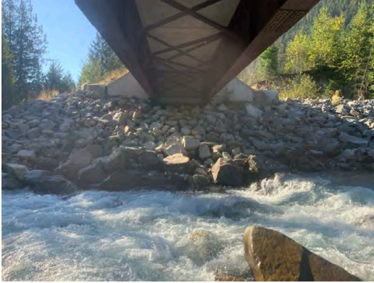
Right Bank Abutment when facing downstream
