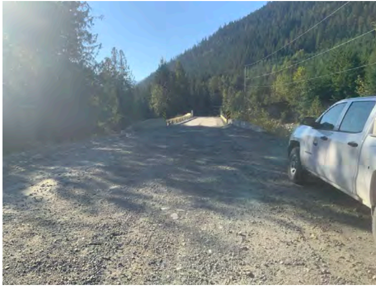
Approach from Left Bank when facing downstream
